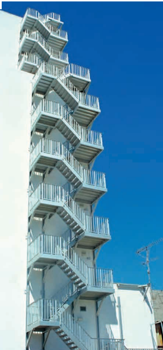
Stair suspended from the façade
