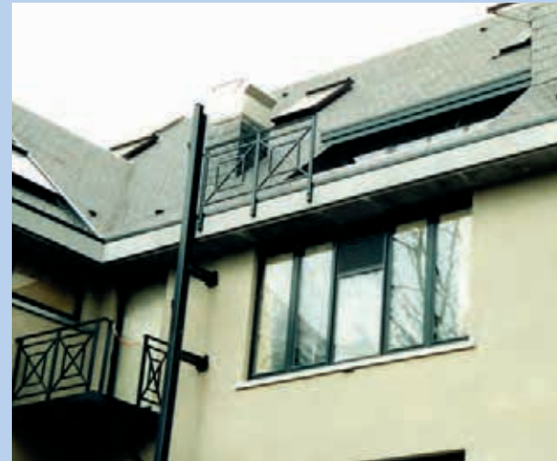
Guardrail with custom design
