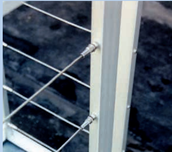
Guardrail using stainless steel cables
